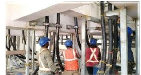
EHV UG Cable Works
